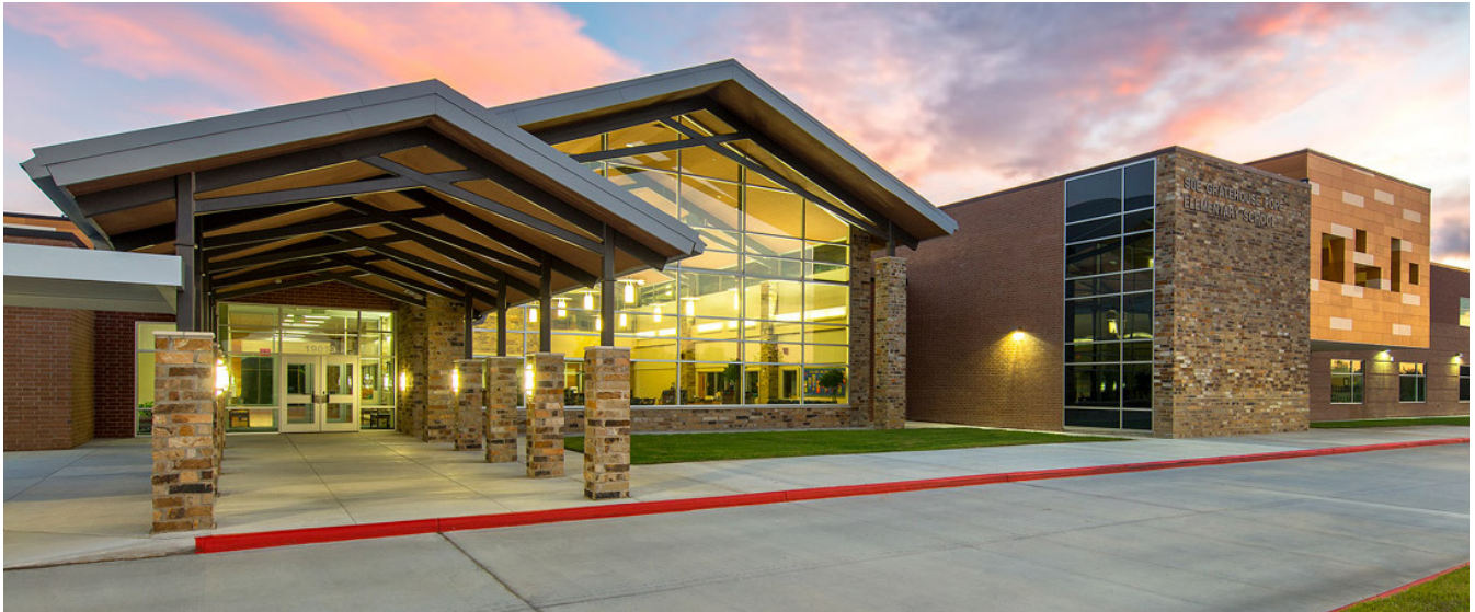
Pope Elementary School – Cypress-Fairbanks Independent School District, Harris County, TX
